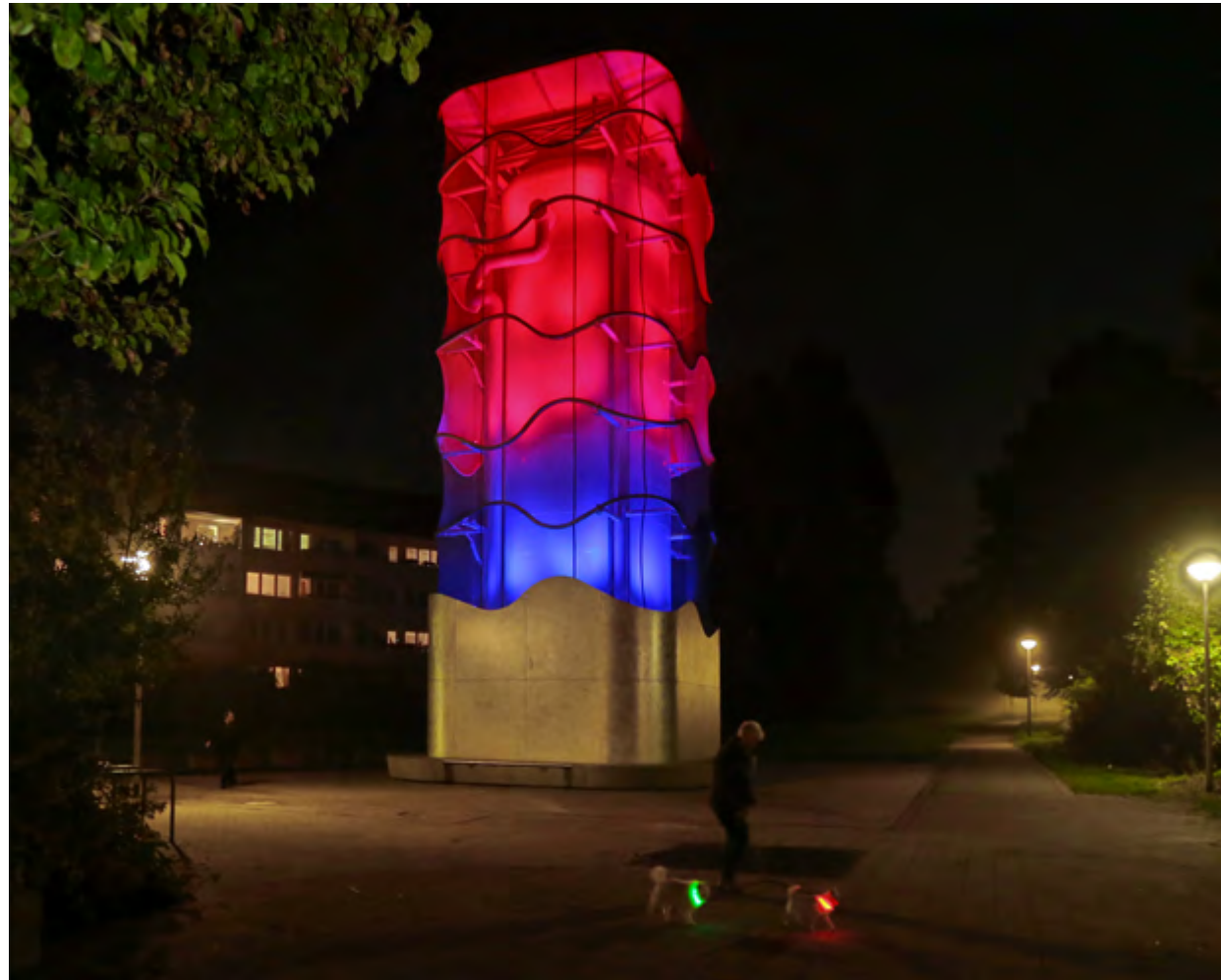
Architectural integration of a district heating water storage tank in Hildesheim. Lighting colour fades from red to blue according to the amount of energy stored in the tank. ©Lighting design
